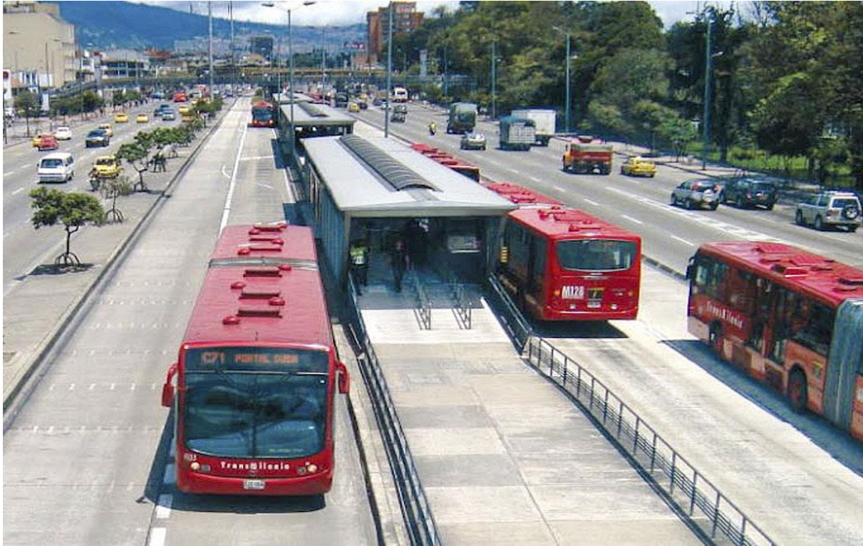
Bus Rapid Transit (BRT) (Trans Milano) Bogota / Colombia
